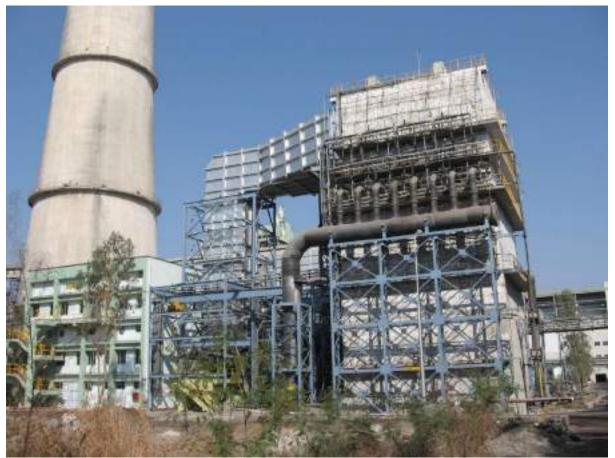
(India's first Sea water FGD system with 100% of flue gas, for 2 X 250 MW DahanuTermal Power Station at Dahanu, Maharashtra, India installed by Ducon)
