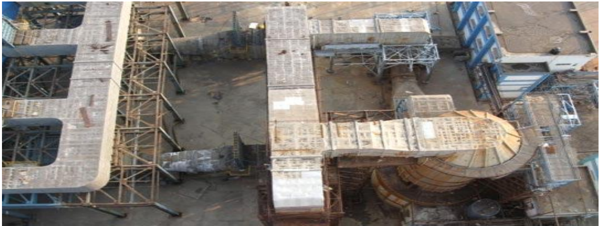
(India's first Wet limestone FGD system on coal fired power plant with production of saleable Gypsum for 2 x 600 MW Udupi Thermal Power Station, Karnataka, India. installed by Ducon)
