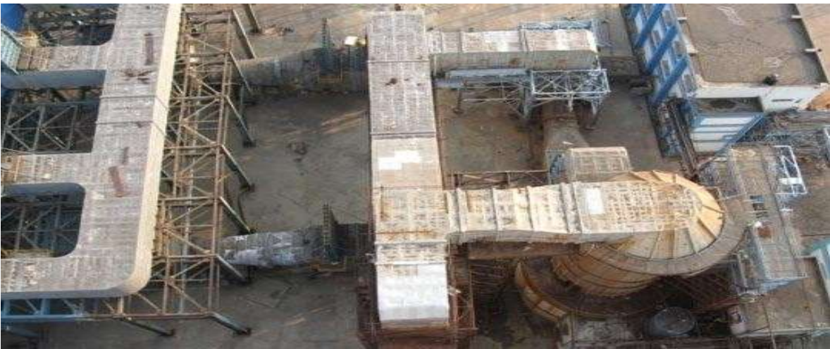
(India's first wet limestone FGD system on a coal-fired power plant with production of saleable gypsum for 2 x 600 MW Udupi Thermal Power Station, Karnataka, India, installed by our Company.)
